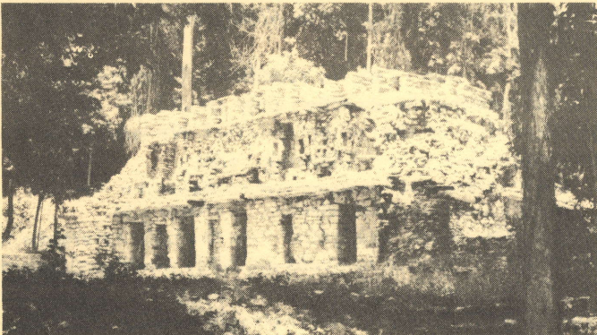
Fig. 14—Structure 19 Yaxchilan. Before restoration (after Maler 1901-1903) and after restoration.
